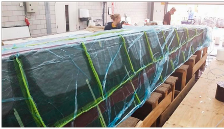
Fig. 14: Bridge beam during vacuum injection
