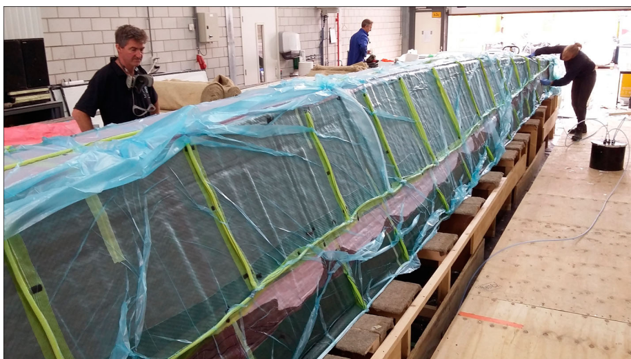
Fig. 4: Production of the 14m long bridge
