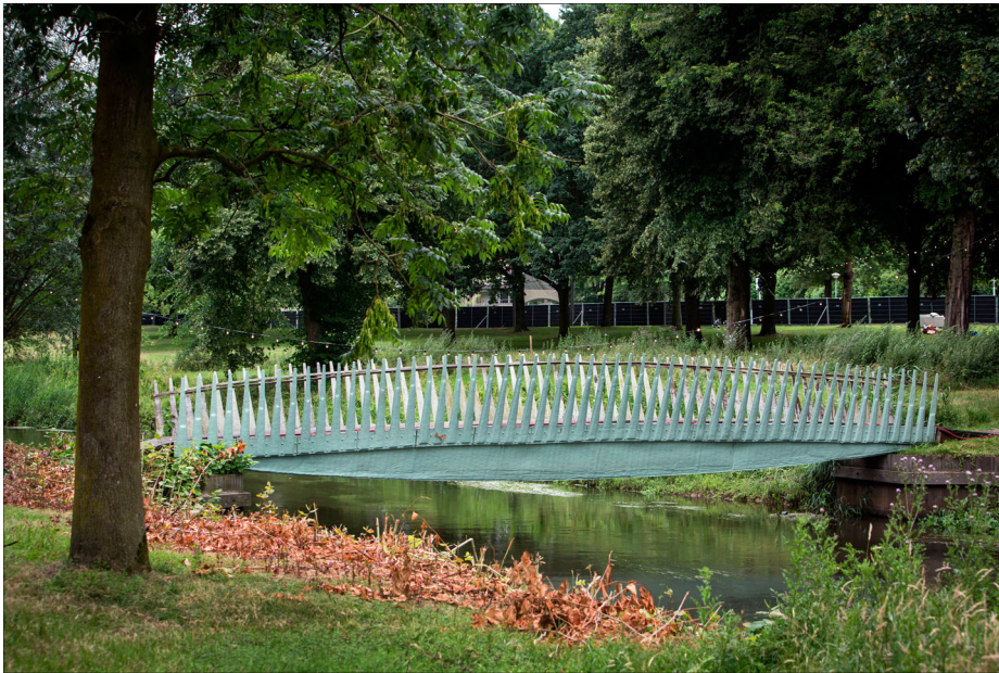
Fig. 1: The bio-composite footbridge, 18 months after the installation across the river Dommel
