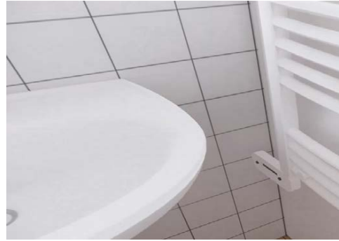
Figure 2: Video still of access to the heating control. Link to video:
