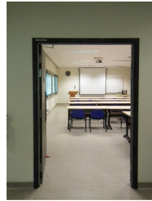
Fig. 3. Full color image of a typical door showing large contrast of color with the surrounding walls and a continuous color defining the three sides of the door.
