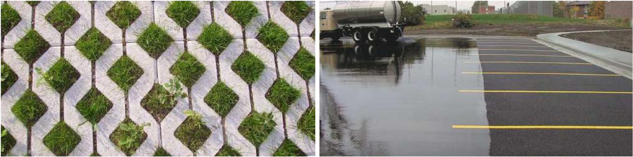
(a) Permeable pavement with grass to increase water absorbance (TreelineHomes, 2016). (b) Difference in runoff between permeable and non-permeable asphalt (CivilOgistix, 2017)
