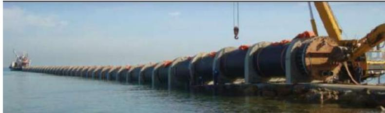
**Figure 6.59:** Positioning the outfall for the final section
