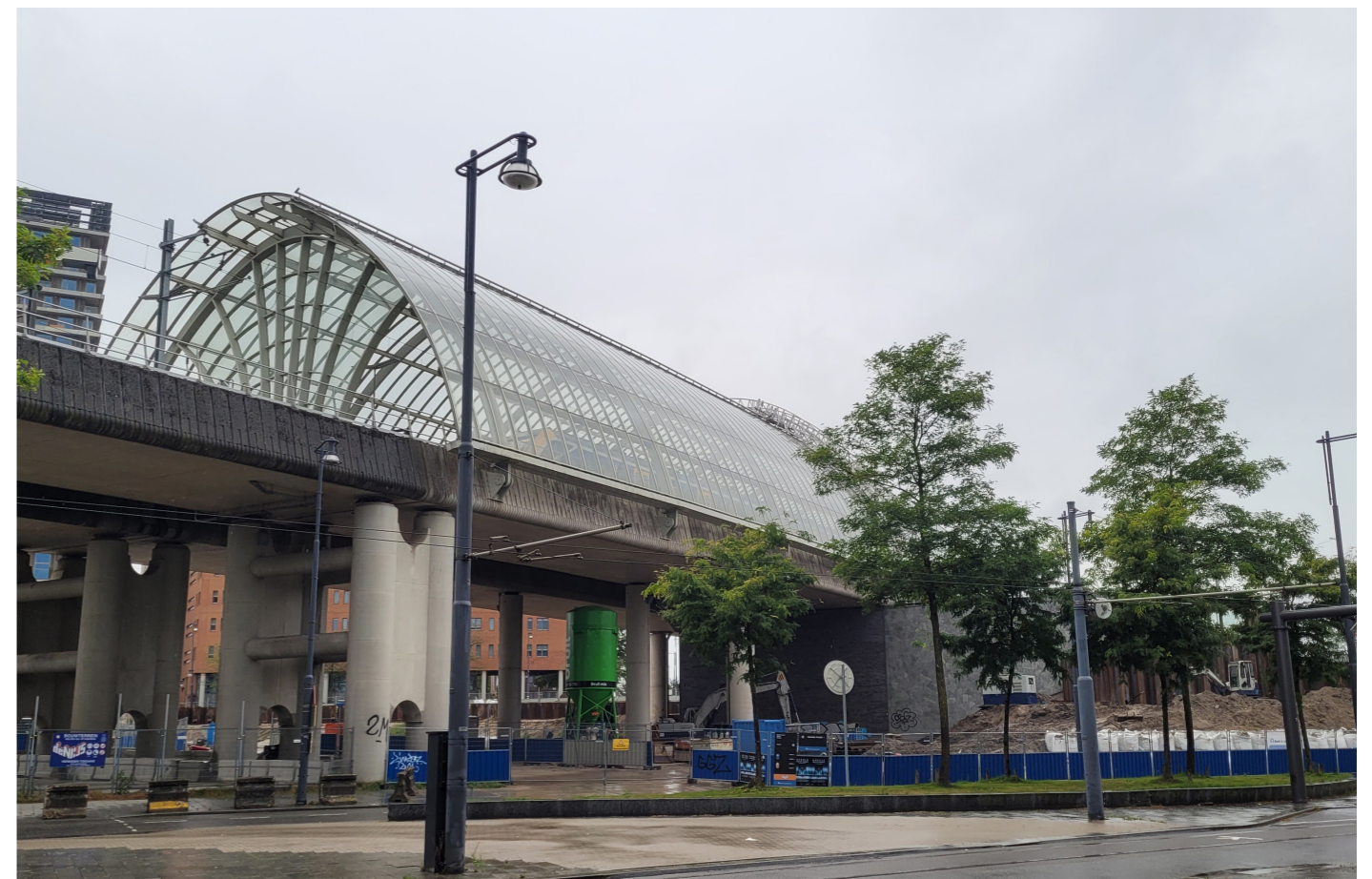
Photo A.3.2: Impression of infrastructural barriers in Sloterdijk Station Area
