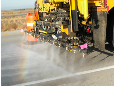
Figure 2.5: Topical application (spraying) of LiNO 3 solution to an ASR affected pavement [49].
