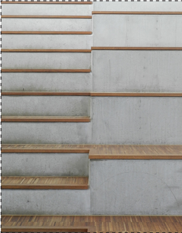
Figure 14 - Double use of the staircase Photographs by Author (2018).
