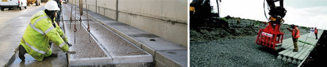
Figure 5.5: Applying concrete in infrastructure projects in the Netherlands (Diemel & Fennis, 2018).
