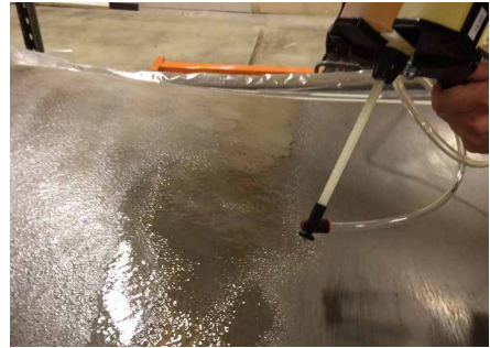
FIGURE 6.15 Applying the hard coat
