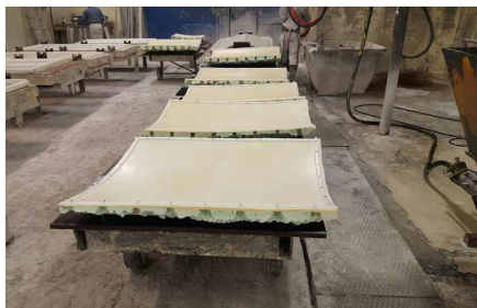
FIGURE 6.30 Intermediate moulds for ring 3-9 of the thin-walled GFRC hyperbolic shell before the first casting.
