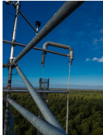
(b) At the top of the tower, the fiber is led through a bend made of PVC and padded with foam.
