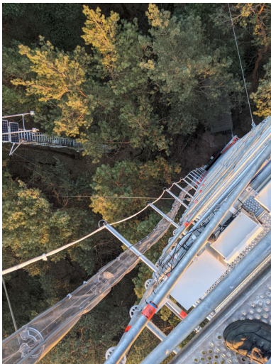
(c) The sun screen (gray mesh) around the bare cable and the cable with a cotton sock run parallel to each other up the side of the tower.
