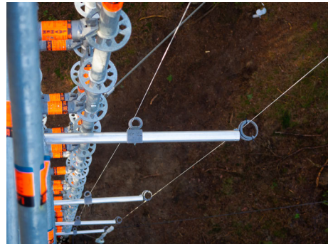
(d) The metal arms hold the wet fiber (outer) at 0.90 m from the tower, and the dry fiber (inner) at 0.45 m from the tower. The lower levels of the tower (up to 20 m) have an additional support column at 0.35 m from the platform edges.
