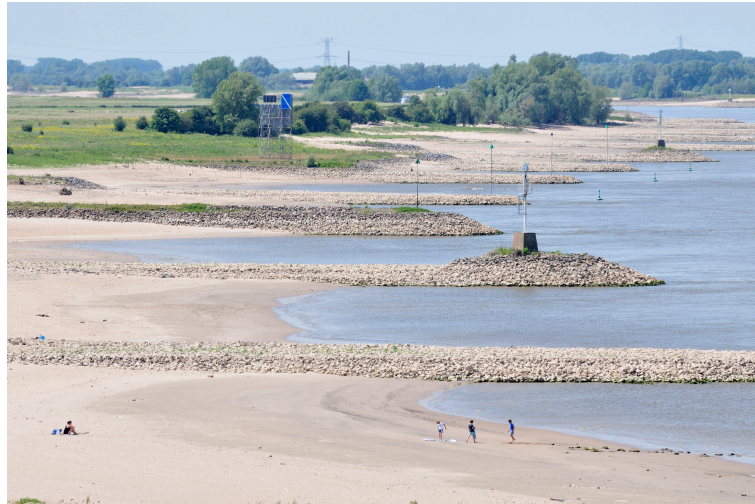
Figure E.2: Groyne field beach along the Waal appearing during low water conditions (Van Lokven, 2011)
