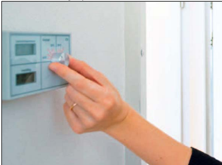
Figure 4.8b. Manual thermostat before installation of the Energy Monitor
