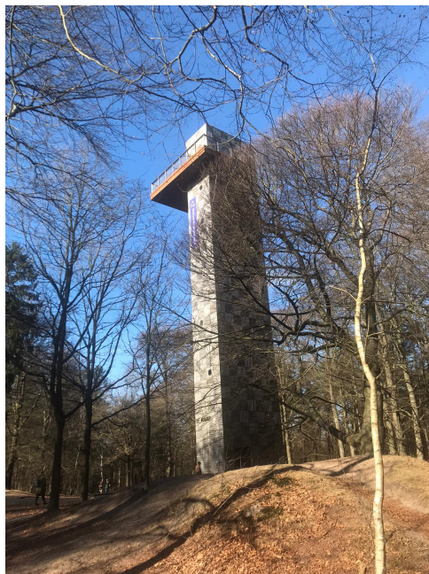
Figure 7.11: The viewpoint for the receiver location. The tower is higher than the treetops.
