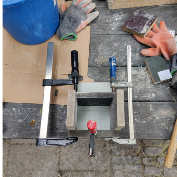
Step 7 / The soil should be built up in layers within the formwork. This is very important, my first test I compacted everything at once, making it very brittle and non-compacted.
