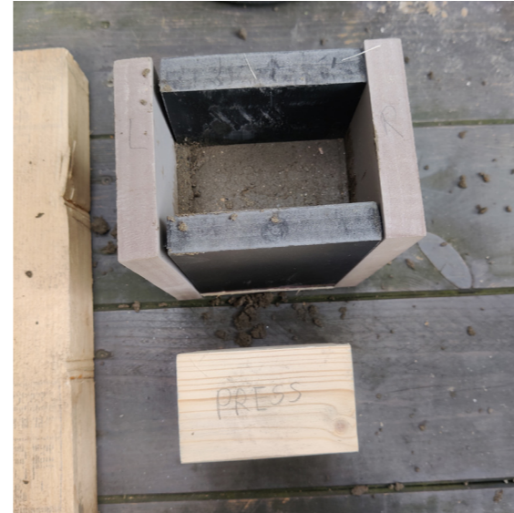
Step 8 / Ramming should be carried out systematically, ramming along the sides first, constantly crossing from side to side to obtain an even result, then ramming the centre until the entire layer is dense and hard.
