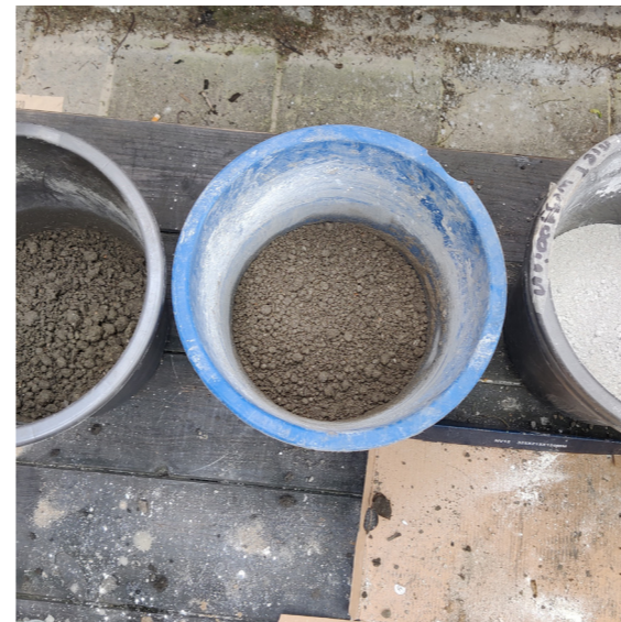
Step 2 / Mix the dry elements well before adding water.
