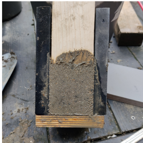
Step 10 / Gradually add and compact Repeat the ramming steps until you have reached the desired height.
