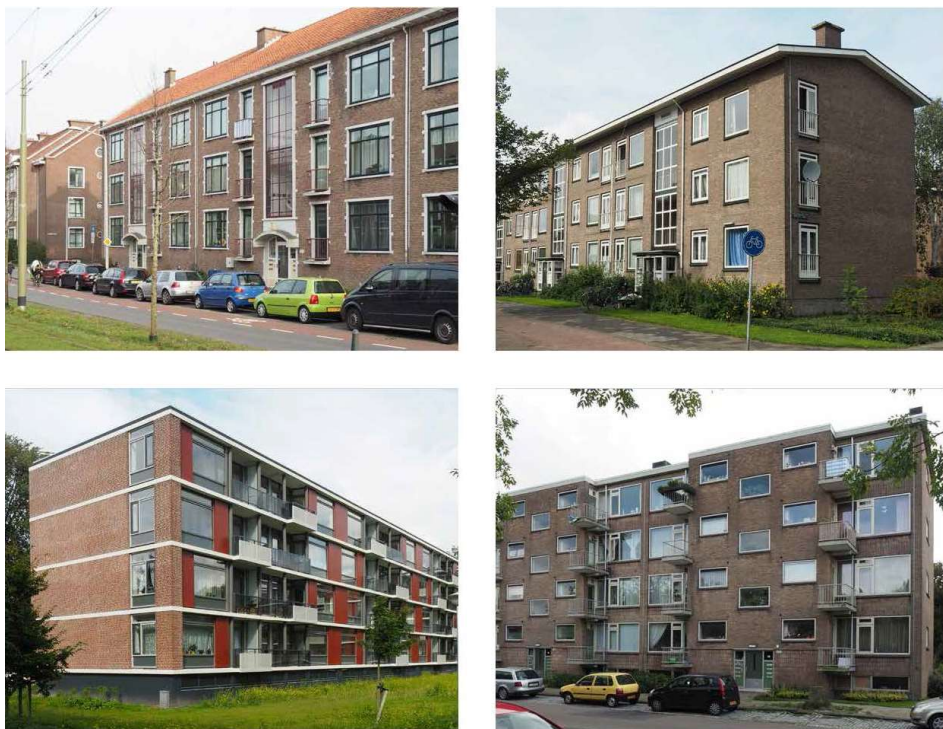
Figure 5. Walk-up apartment buildings in Den Haag owned by housing associations. The change in architecture was the consequence of directives from the ministry about reducing cost by avoiding expensive materials (ceramic); a lack of skilled labour; and new ideas about modern architecture, standardisation, and industrialisation. Top pictures involve early postwar architecture from the neighbourhood Moerwijk, and bottom pictures show late postwar architecture from the neighbourhood Mariahoeve. The pictures on the left involve the Muwi construction system, and the pictures on the right show the Korrelbeton system. Only in some specific cases (Airey, Coignet) is there a clear relationship between architecture and construction system. Pictures by Leo Oorschot.
