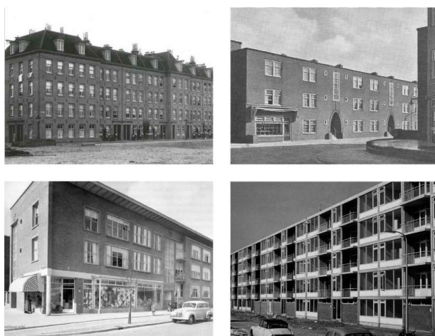
Figure 3. Four subtypes. Top left: subtype 1 interwar traditional construction methods Amsterdam. Top right: subtype 2 interwar traditional construction methods Den Haag. Bottom left: subtype 3 postwar mixed construction methods. Bottom right: subtype 4 postwar construction systems. Pictures are from the municipal picture data banks of Den Haag Amsterdam and Utrecht.
