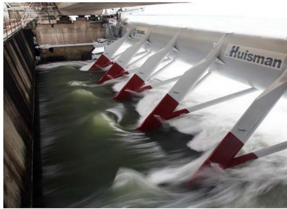
Figure 1.1: Turbines in operation in the Eastern Scheldt barrier (Leopold & Scholl, 2019)
