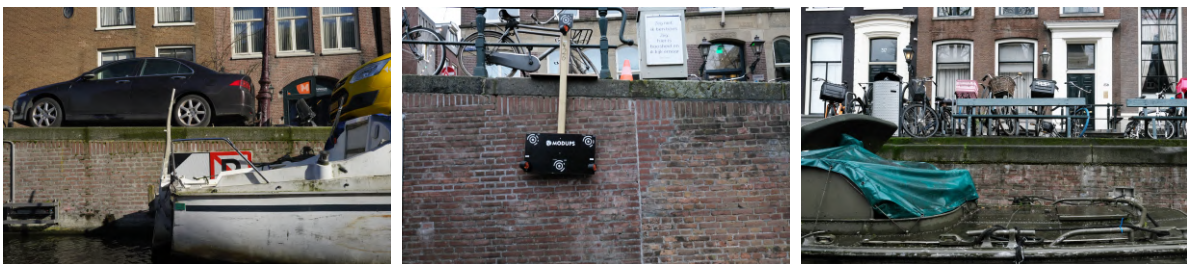
Figure 3.1: Three example images of quay walls are depicted to illustrate the complexity and variety within the scene. This complexity includes variations in scene lightning, camera position or quay wall textures. Furthermore, the images often contain partial occlusion by for example boats, signs or ropes.
