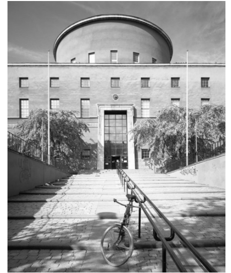
(Descending): Fig. 24. Stockholm City Library entrance portal, RIBA archival photograph (1987), Chris Martin; Fig. 25. Stockholm City Library entrance portal analysis, Sketch, NTS.
