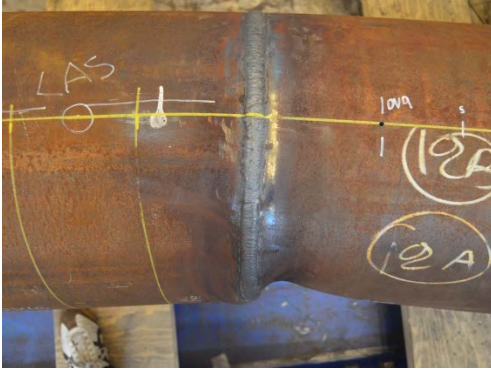
(a) Unpressurized specimen T8 (right side of the fault)
