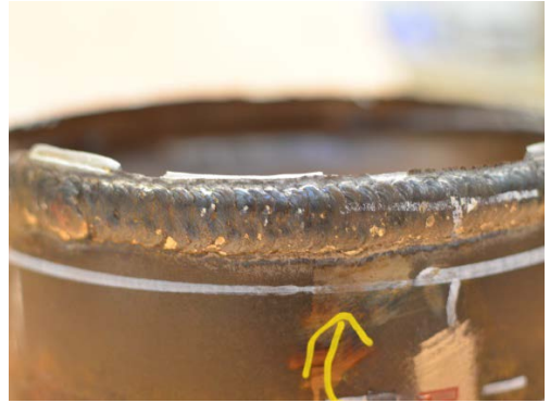
(b) Close-up of rupture surface near weld
