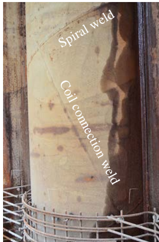
Figure 4.2 Coil connection weld in a spiral-welded tube applied in a combined wall.
