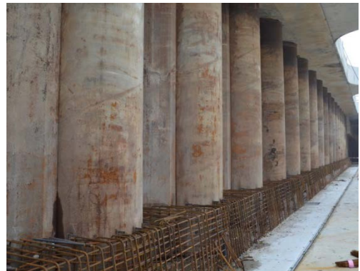
(b) Exposed combined walls in building pit
