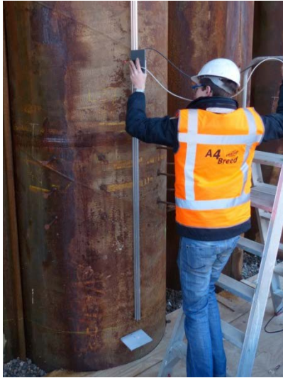
(b) Measurement setup in operation
