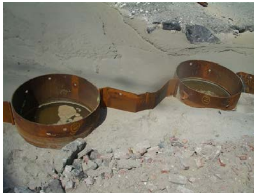
Figure 4.4 Example of a combined wall system under construction (ArcelorMittal, 2008).
