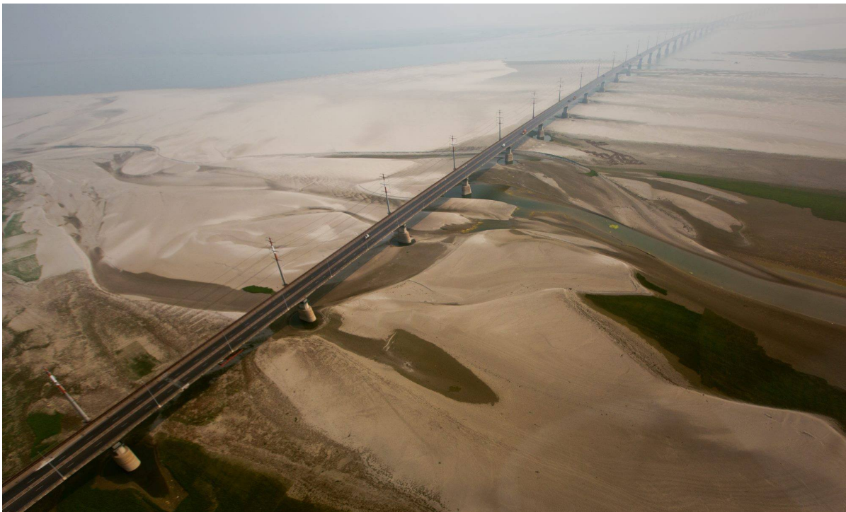
Fig. 4.16 Aerial photograph of the Bangabandhu bridge, providing an indication of the high (seasonal) sedimentation rates. By Paul (2015).
