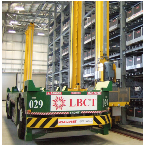
Figure 2.5: Electric AGVs can be charged by swapping out their depleted batteries in battery swapping stations[9]
