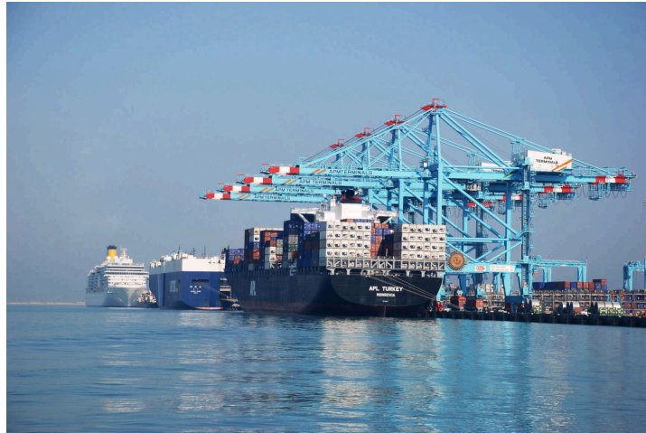
Figure 1.2: APM Terminals Bahrain operating within the Khalifa Bin Salman Port of Manama, Bahrain [46].
