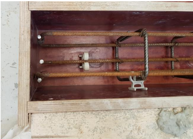
Figure 3-25: Top view with spacers for reinforcement mesh
