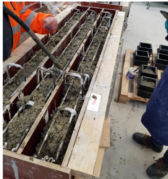
Figure 3-34: Vibrating the concrete
