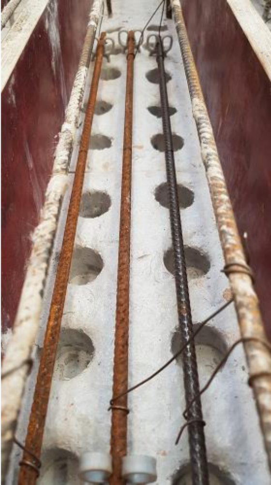
Figure 3-30: Coupling reinforcement
