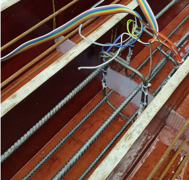
Figure 3-26: Stirrup at the joint
