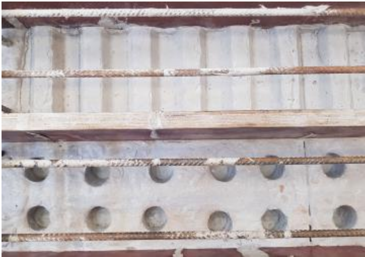
Figure 3-32: Profiled and holed interface
