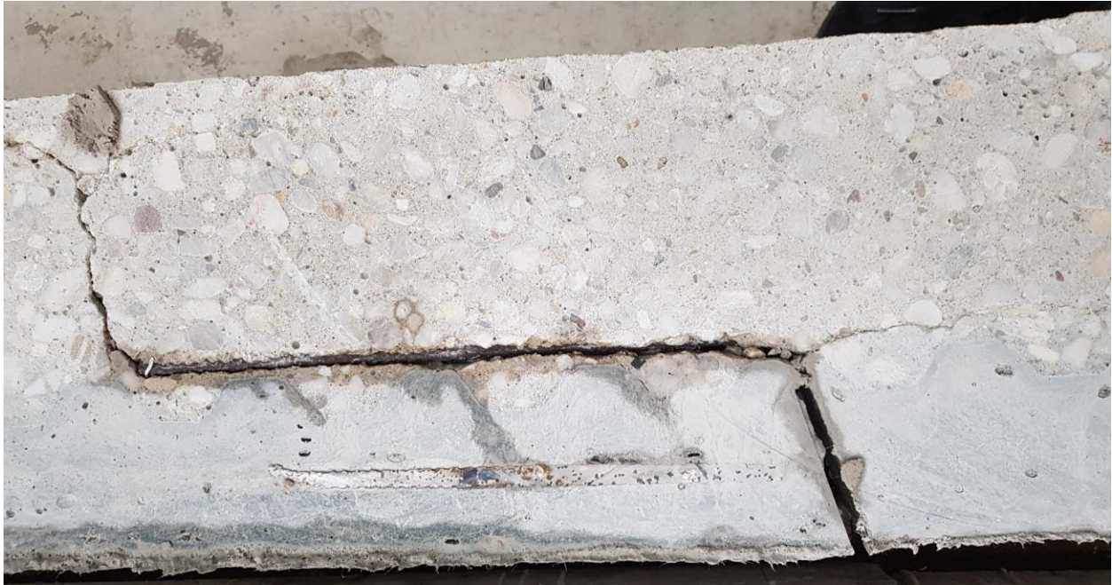
Figure 3-130: Crack propagation of the sample with a profiled interface
