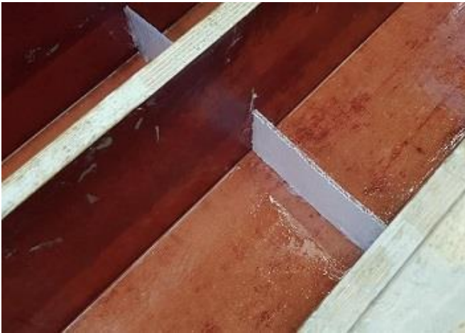
Figure 3-23: Joint in the middle of the beam glued with kit
