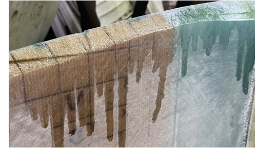
Figure K.2: Treating edge with pure epoxy
