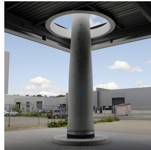
Figure 8.3: Signpost blade foundation (Superuse, 2014)
