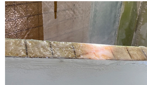
Figure K.3: Treating edge with epoxy aerosil mix
