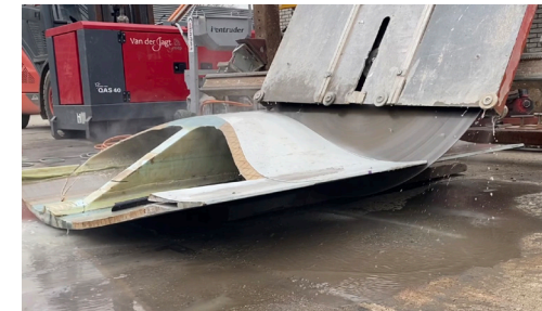
Figure K.1: Cutting the segment using a large circular saw
