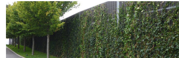
Figure 11.5: Overgrown screen (Gramm Barriers, 2022)
