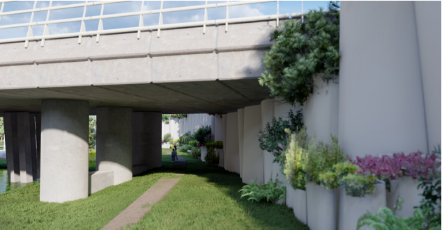
Figure N.4: Blade Barrier integrated with pre-existing bridge structure
