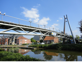
Figure 1: The footbridge in Ninove, Belgium.
