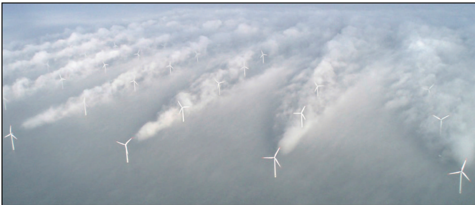
Figure 1.3: Horns Rev offshore wind farm with, normally invisible, wakes. Source: Christian Steiness. See also (Hasager et al., 2013) for more information on the picture.
