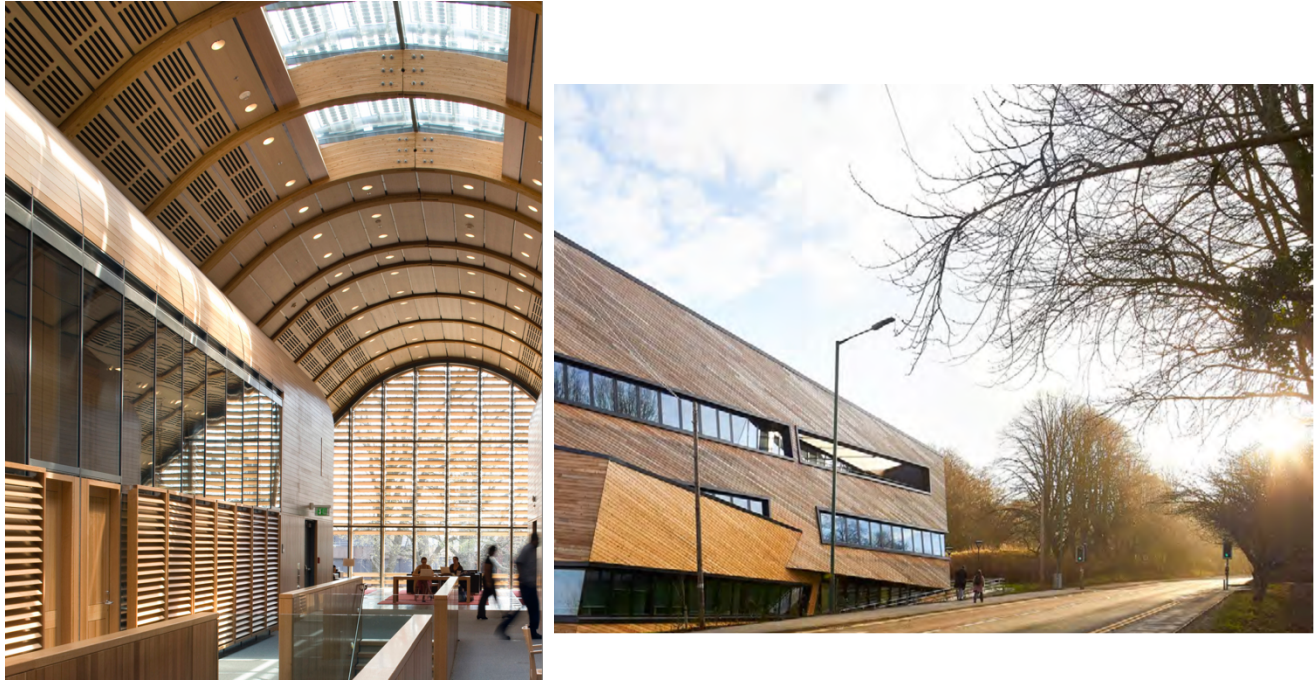
Figure 9.2: Kroon Hall, Yale University (left) & The Odgen Centre for Fundamental Physics (right). Source: Arup 2011
