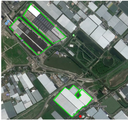
Figure 6.47: Layout of the buildings analysed, the reference point is highlighted in red
