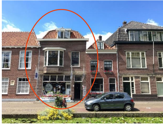
Figure 73 Location for the 3D real life model assessment of the PV + PDLC system
