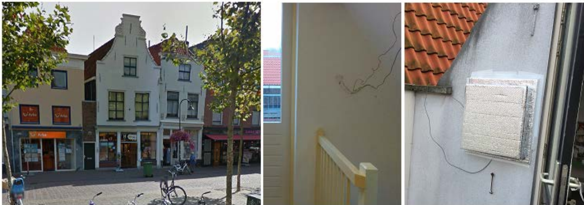
Figure 10.1- Case study 1- The whole building (left), the inside surface of the wall (middle), and the outside surface and sensors covered by the box (right). Location: Delft, the Netherlands
