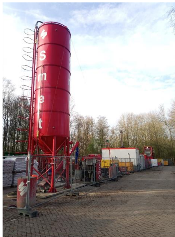
Drilling location DAPGEO-02 (500m)
