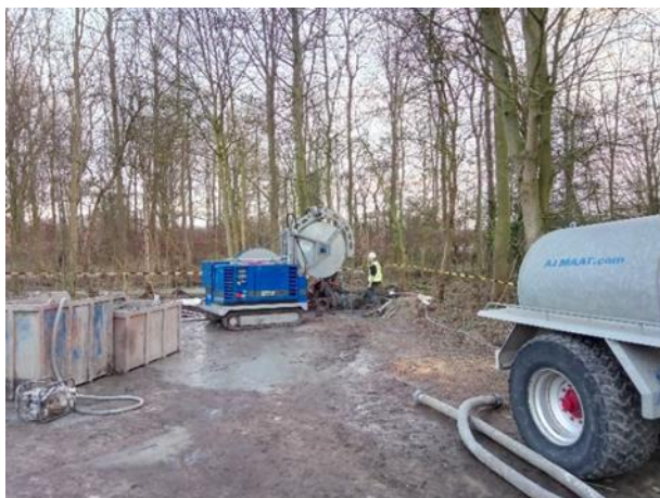
Grouting of DAPGEO-02 (200m)
