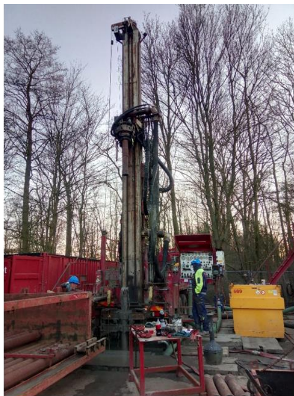
Drilling of DAPGEO-02 (500m)
