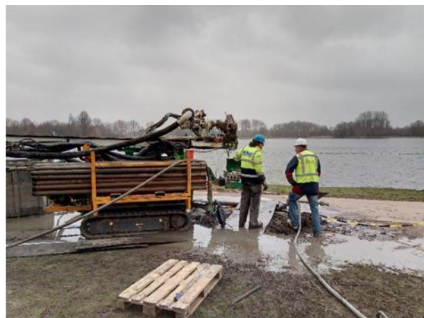
Drilling of DAPGEO-02-01B (50m)
