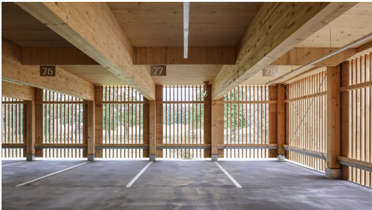
Figure 75. Timber multi-storey car park Bad Aibling (HK Architekten, 2022)
