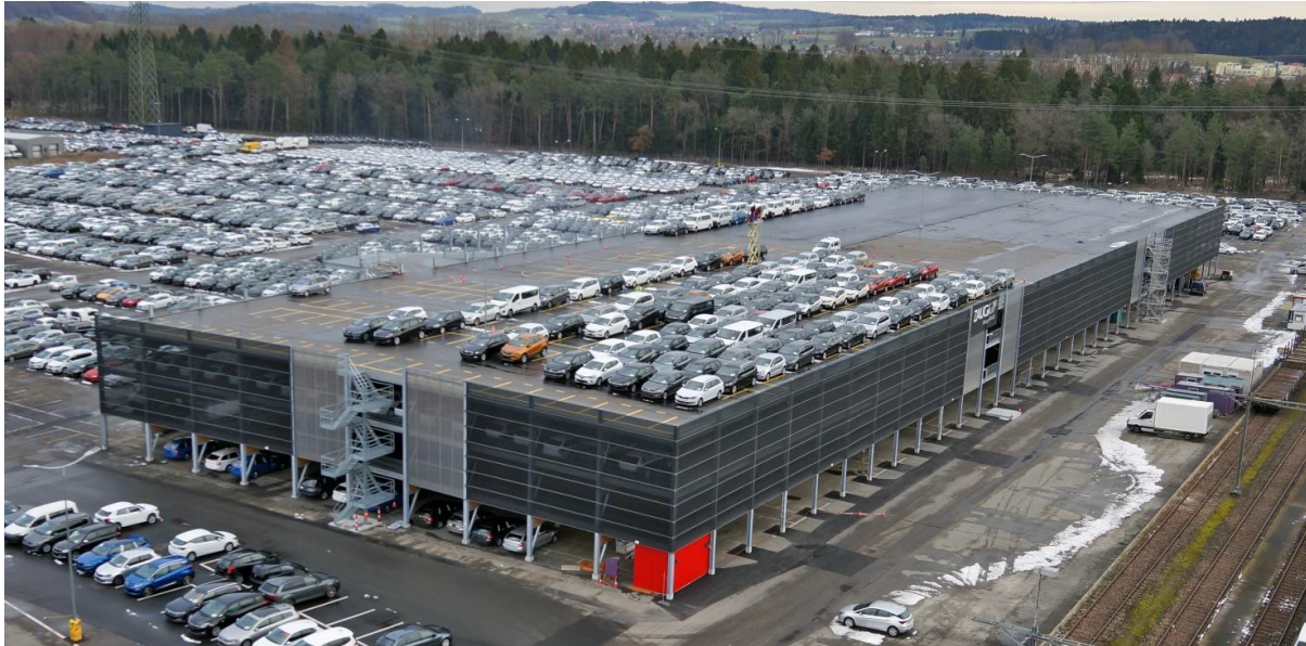
Figure 57. Steel elements in façade of car park (Zaugg, 2018)
