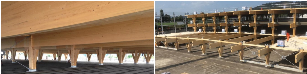
Figure 54. Structure of all-timber car park (Zaugg, 2018)
