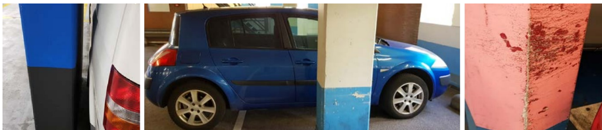
Figure 3. Examples of problematic dimensions of parking bays and location of columns (Van Drooge, 2020)
