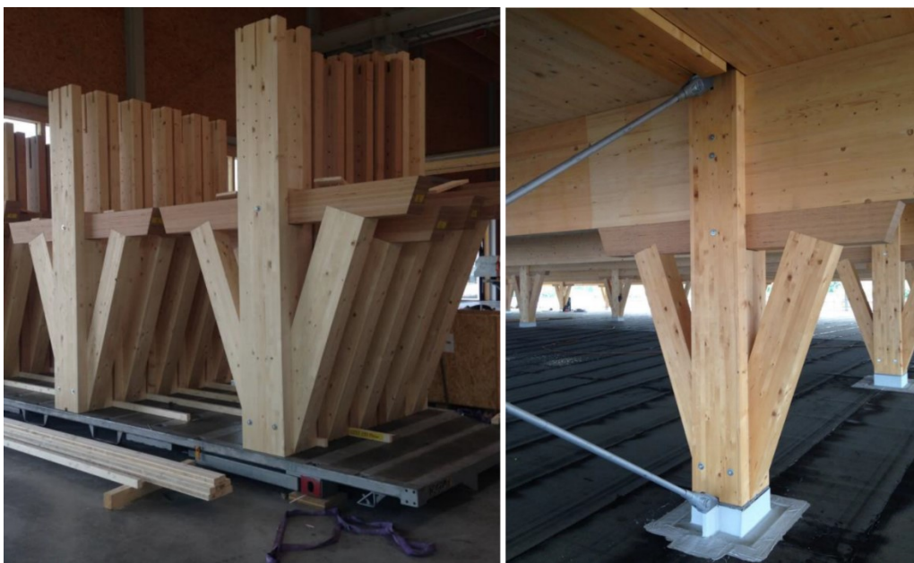
Figure 55. V-shaped columns (Zaugg, 2018)
