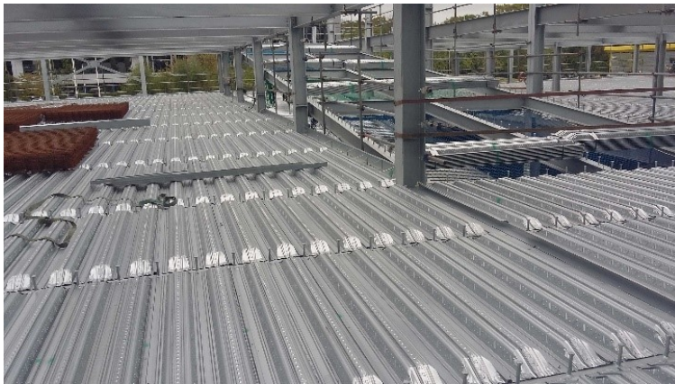
Figure 23. Corrugated sheet metal floor under construction in car park (SMD Ltd, 2019).
