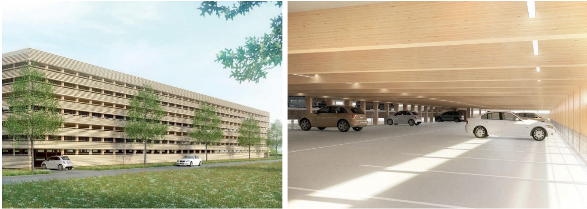
Figure 60. Artist impression of multi-storey car park in BauBuche (Technical University of Munich & Pollmeier Massivholz GmbH & Co.KG, 2015)
