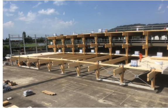
Figure 27. Bin wide girders supporting perpendicular floor elements framing system (Zaugg, 2018).
