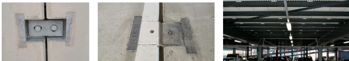
Figure 32. Left & middle: Couplers between deck panels to create horizontal stabilizing element. Right: Diagonal bracing as horizontal stabilizing system (Park4all, 2019a).
