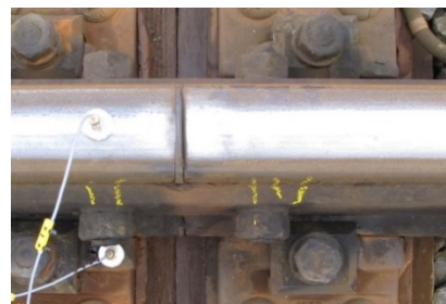
(e) IRJ number 7 with rusty fastening.
