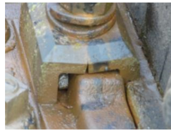
(h) IRJ number 9 with a crack in the fastener, side view.
