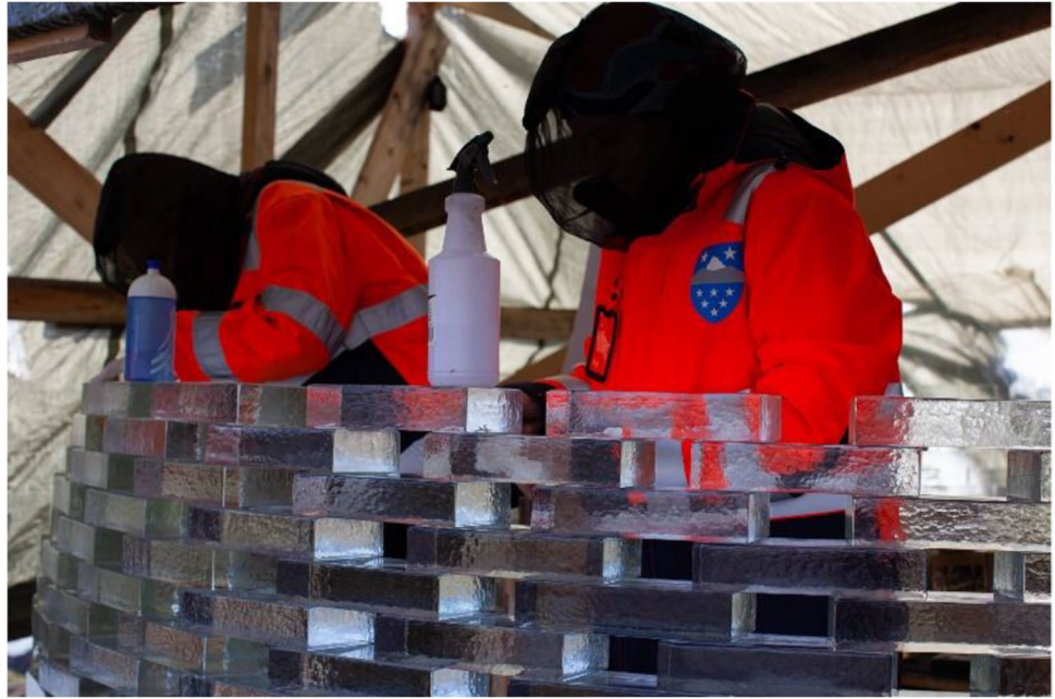
Fig. 21 The two TU Delft researchers bonding glass bricks on-site. Besides the adverse climate conditions, mosquitos proved to be an equal challenge in Greenland, deeming the use of mosquito nets necessary
