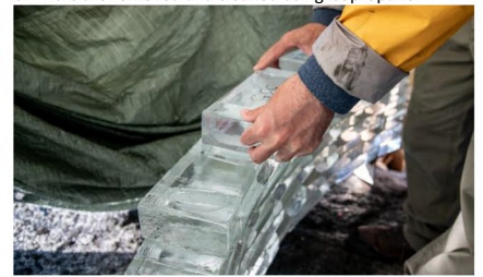
8. Placement of brick using manual pressure
