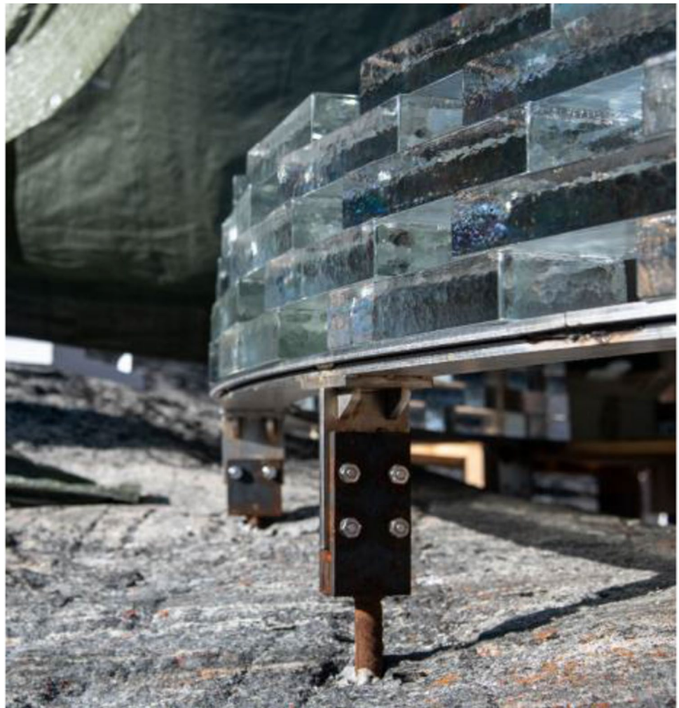
Fig. 22 Foundation of the glass-brick Qaammat Pavillion
