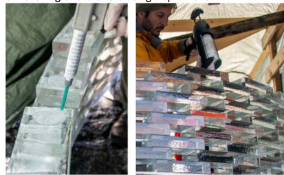
7. Dispensing of 3M DP610 (left) and of the Fast-curing experimental Dowsil Adhesive (right).
