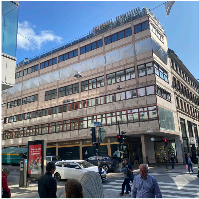
Bradenberg Department Store under renovation
