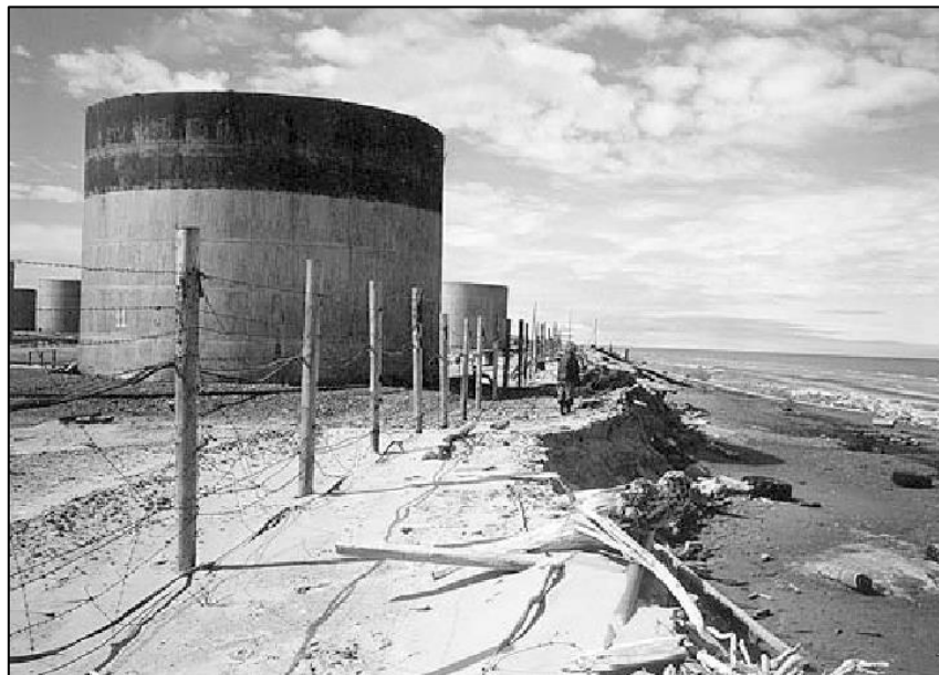
Figure 1 Varandei oil terminal at risk by wave-cut cliff on the coast of the Pechora Sea Ogorodov (2005).
