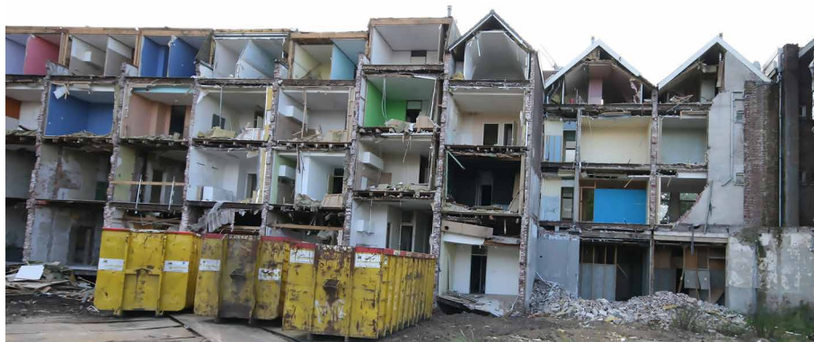
FIG. 2.6 Klushuizen (DIY-houses) in Rotterdam, the Netherlands [Source: Klushuis.Wordpress]
