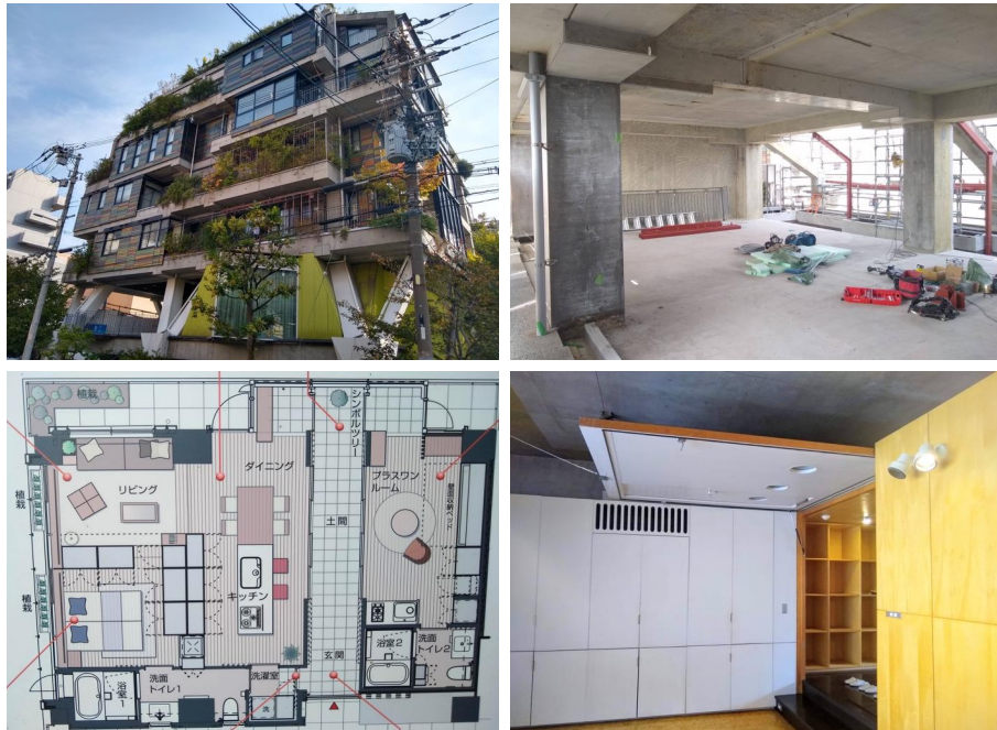
FIG. 2.4 Clockwise from above left onwards: the NEXT21 complex; Open support structure before infill renovation; Unit 303 'Independent Family House' with open partition wall; Floor-plan of Unit 501 'Plus One House' [Source: Bob Geldermans]
