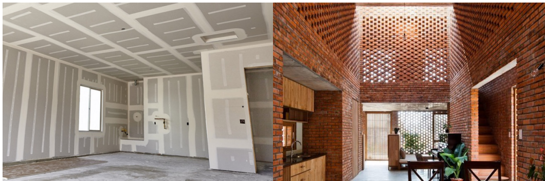
FIG. 1.10 Conventional plasterboard partitioning (left) and a modern elaboration of brick partitioning [Source: Shutterstock/Dezeen Magazine]
