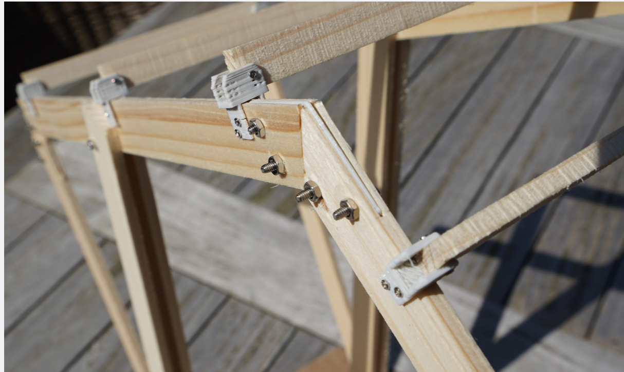
figure 06 - Roof beam joint
