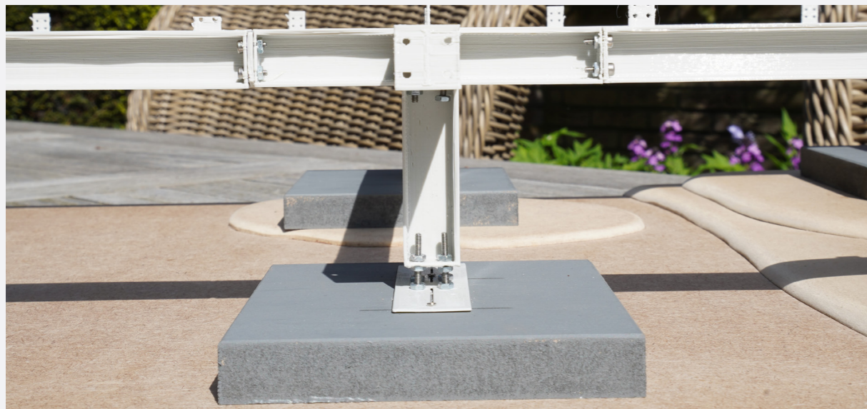
figure 22 - Overview of Central Heart foundation structure
