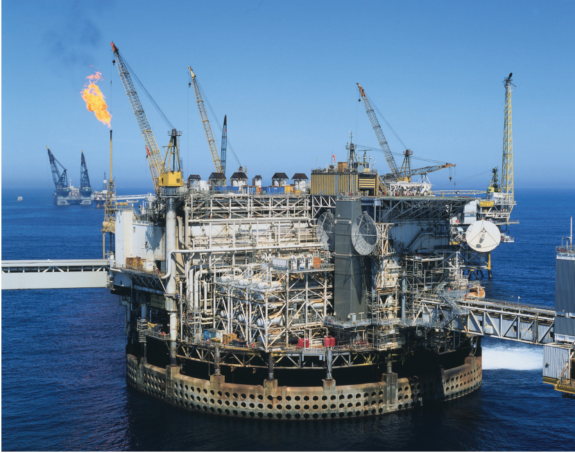
FIGURE 6.3 Ekofisk storage tank. Source: Norwegian Petroleum Museum.
