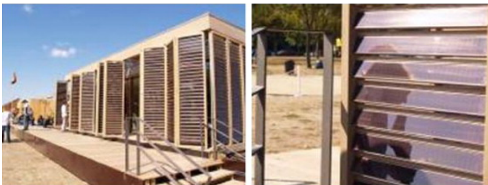
Figure 1.4: PV integrated blinds by Technische Universität Darmstadt at Solar Decathlon 2007 in USA [3]
