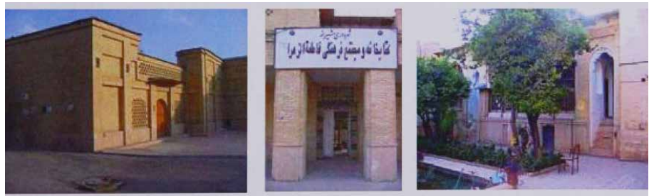
FIGURE 4.19 Neighbourhood library and cultural centre (right and middle) and the local Haj Mohammad Rahim Mosque (left) which have been restored by Fars Urban Development and Revitalisation Company (left). Source: (Izadi 2008, p 219)
