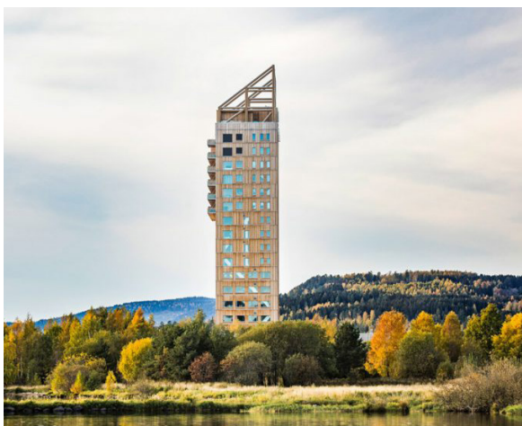
Figure 1.6: Mjøstårnet, Brumminndal by Vollark (2019) Source: http://vollark.no/portfolio_page/mjostarnet/
