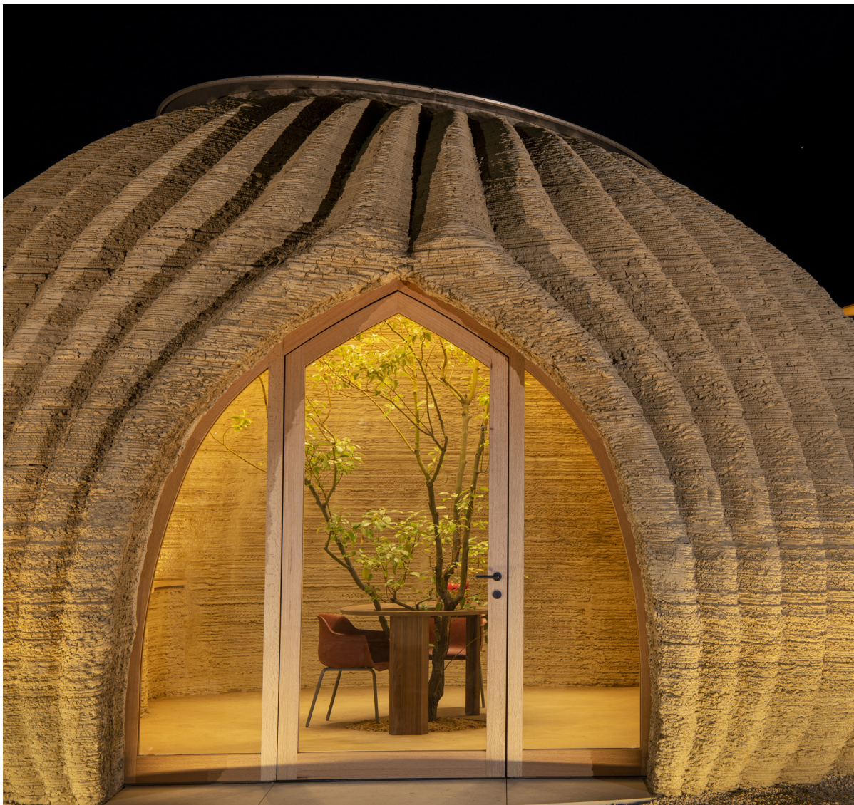
Figure 2.5: Tecla house, engineered by WASP & designed by Mario Cucinella (2021) Source: https://www.3dwasp.com/en/3d-printed-house-tecla/
