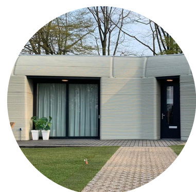
Figure 7.3: Flat window frame connected to 3D printed concrete house, Eindhoven 2019 Source: https://www.3dprintedhouse.nl/en/project-info/project-milestone/
