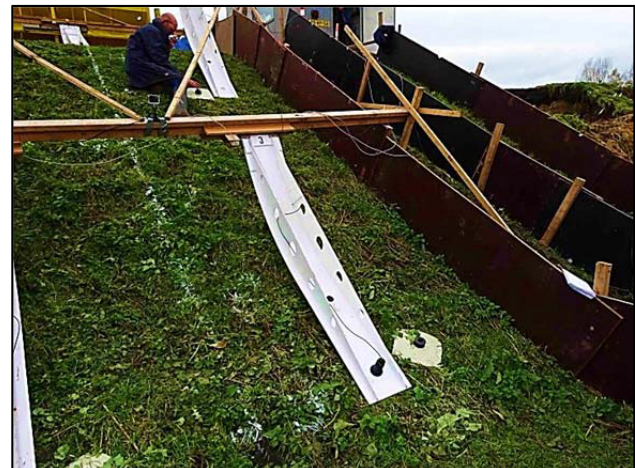
Figure 2. Setup for performing hydraulic measurements during wave overtopping tests.
