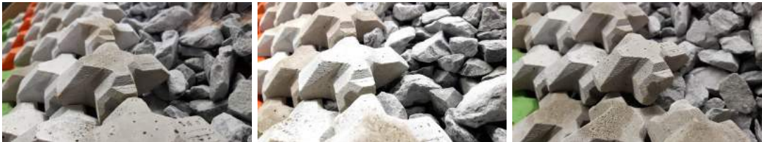
(a) Correct placement (b) Negative fluctuation: tail unsupported (c) Positive fluctuation: wing unsupported
