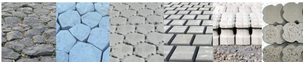
Figure 2.11: Examples of placed blocks: Basalt, Basalton, Ronaton, Verkalit (interlocking), Hillblock and Hydroblok
