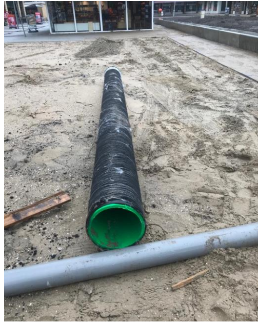
Figure D-2 A Drainage Transport-sewer pipe, made of PVC, with a permeable casing
