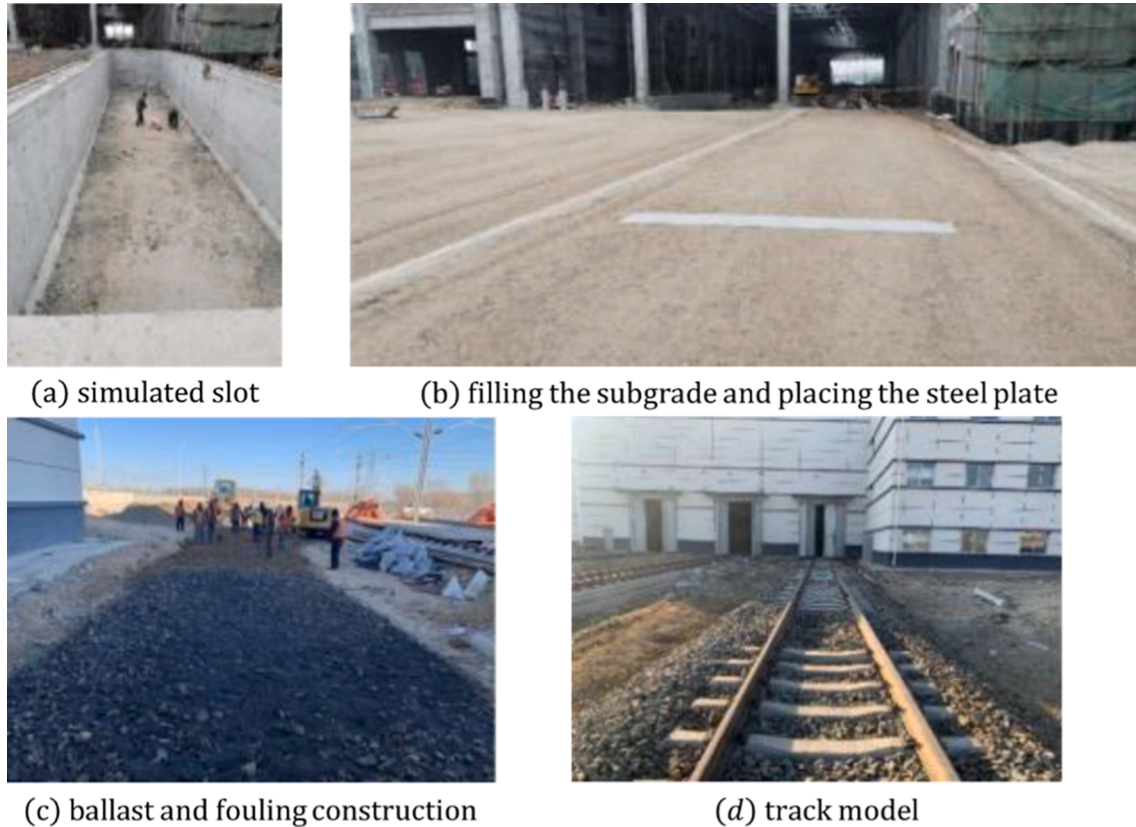
Fig. 3. Full-scale ballasted track construction process.
