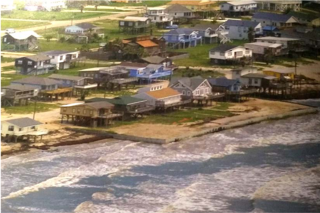
Figure 7. Bulkheads in front of private properties in Galveston Island, west of the Seawall. Source: (Anderson, 2007)
