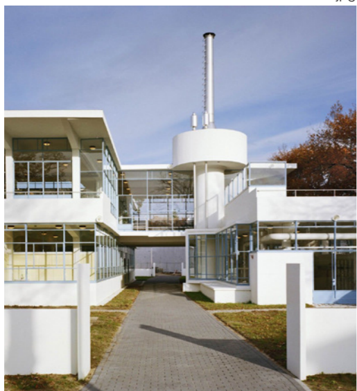
Figure 2: Sanatorium Zonnestraal after transformation by WDJArchitecten, Hilversum, NL. https://i.pinimg.com/originals/8f/b0/a5/8fb0a5bddfd856aaa230626b4e621ec8.jpg
