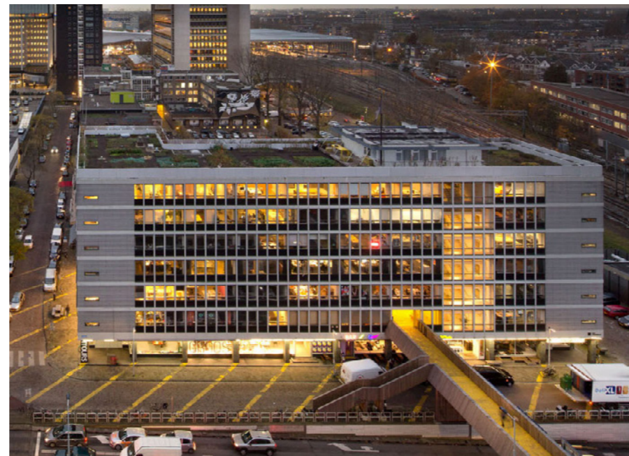
Schieblock (Life back to the building)
