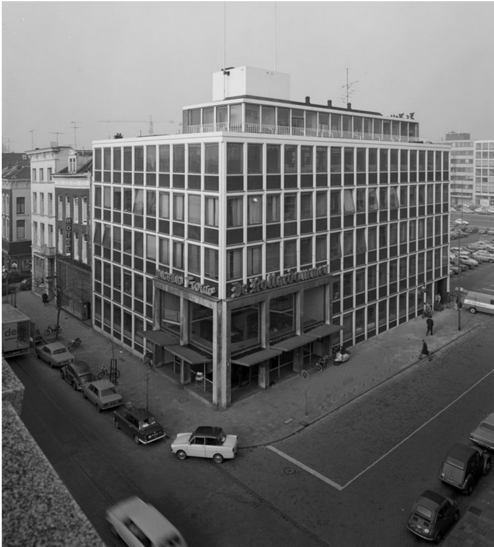
Figure: Photo of the building, 1988.
