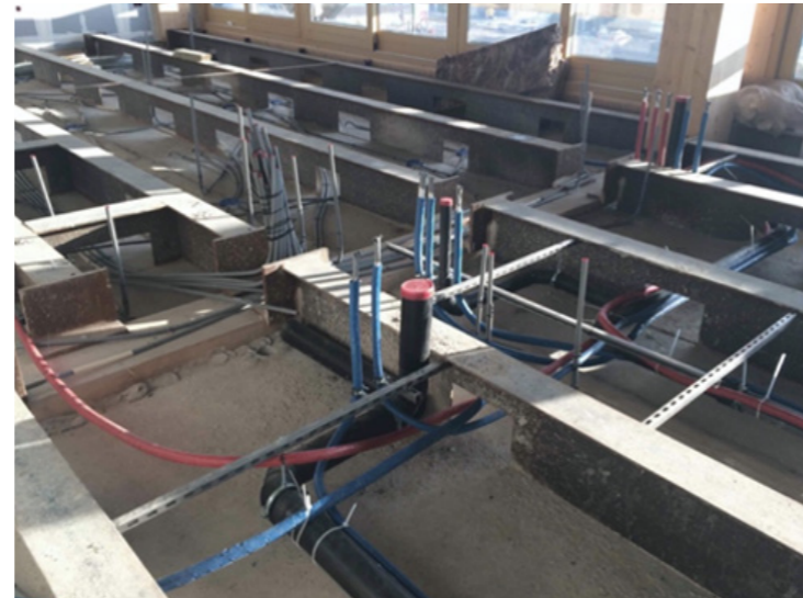
Figure: Hollow Slimline floor system with free positioning of drains and wiring.
