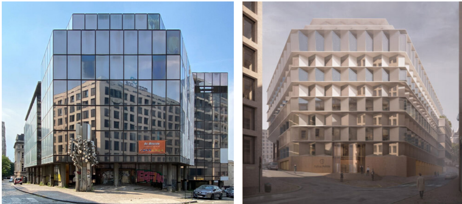
Figure 5: tender project Politiecentrum De Ligne by WDJArchitecten, Brussels. Left - situation before, right - proposal. https://www.wdjarchitecten.nl/projecten/politiecentrum-de-ligne/
