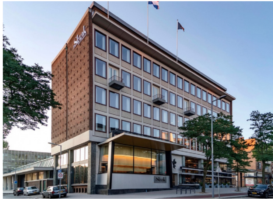
Slaakhuys (approach to preserve the ambience of original)
