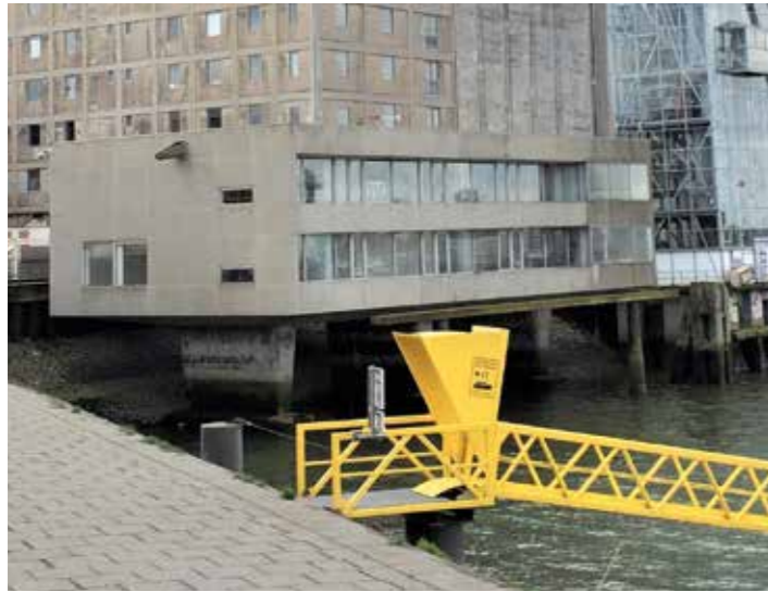
Exterior - north façade
