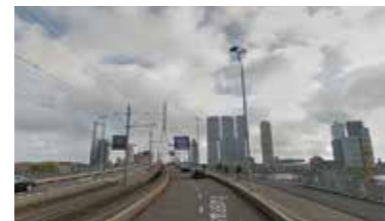
3. Erasmus Bridge, axis in open field
