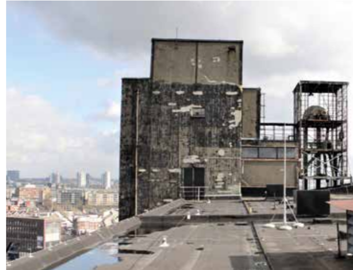
Exterior - west façade
