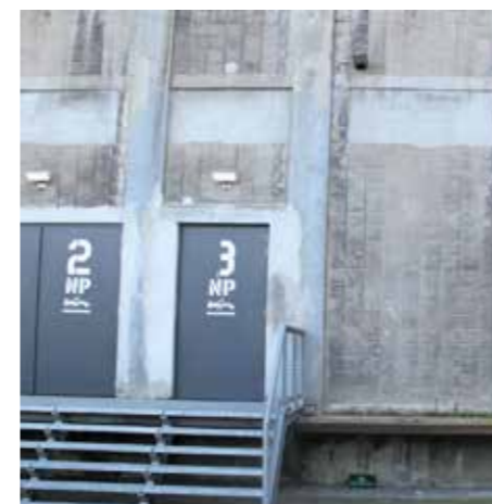
Current - exterior Former façade openings have been filled up with concrete.
