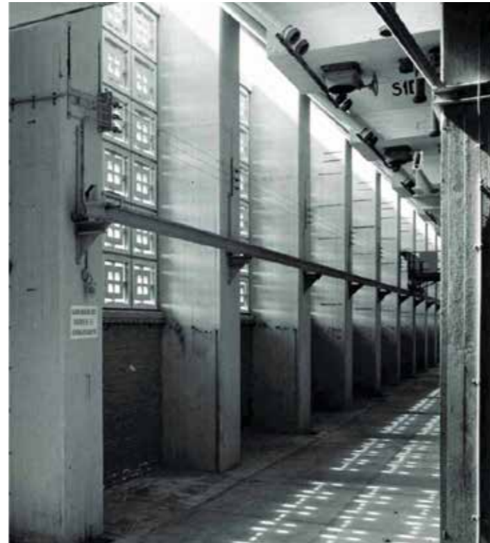
The grainsilo as seen from the Brielselaan (Transformers (2008) Cultuurhistorische verkenning graansilo Maashaven. Rotterdam) Original - interior: daylight coming through plofroosters and creating patterns.
