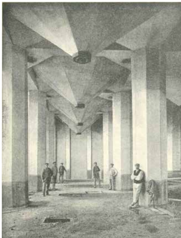
Octagonal silos, Transformerts report, cover
