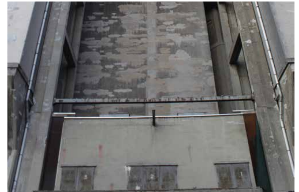
Phase 3 steel beam on which the steel 'Graansilo Mij' used to be
