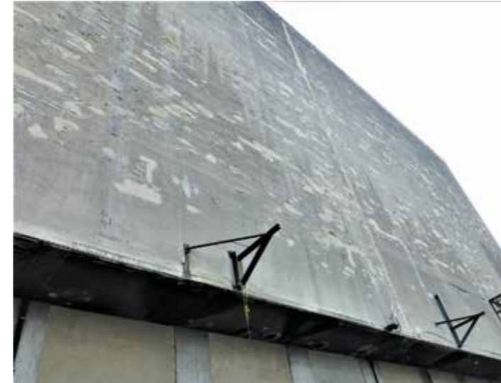
Exterior - north façade
