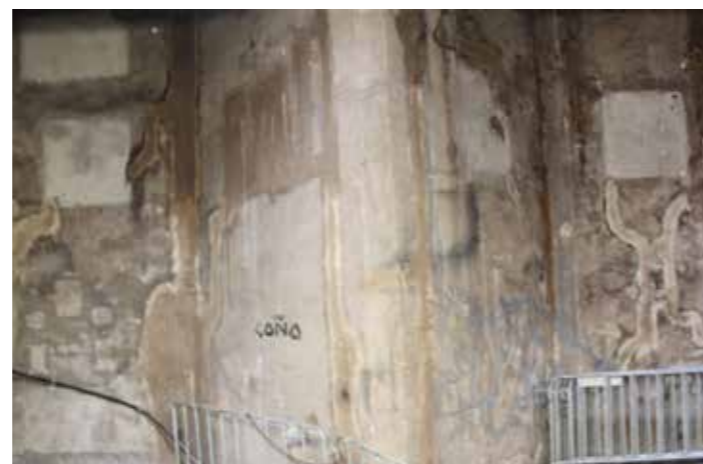
Current - interior Former façade openings have been filled up with concrete.
