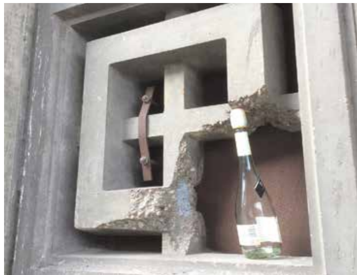
Current - exterior Metal plates visible behind all the plofroosters.
