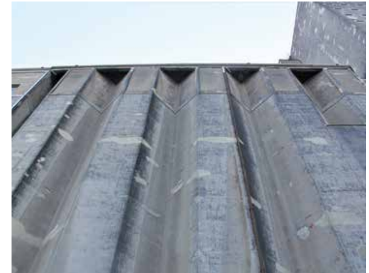
Exterior - northwest façade
