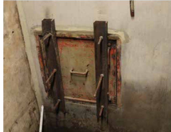
Series of service openings primarily in the basement
