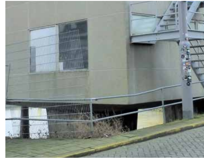
Exterior - west façade
