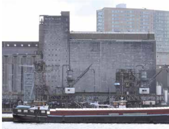
Exterior - north façade
