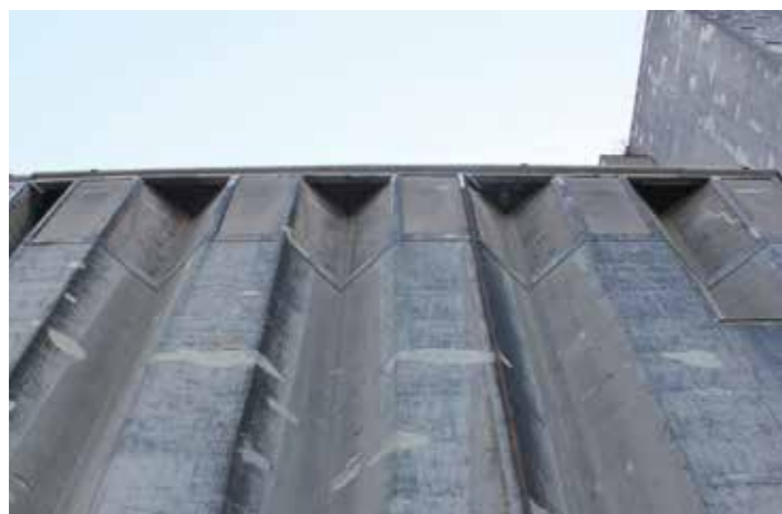
Current - exterior Former façade openings have been filled up with concrete.
