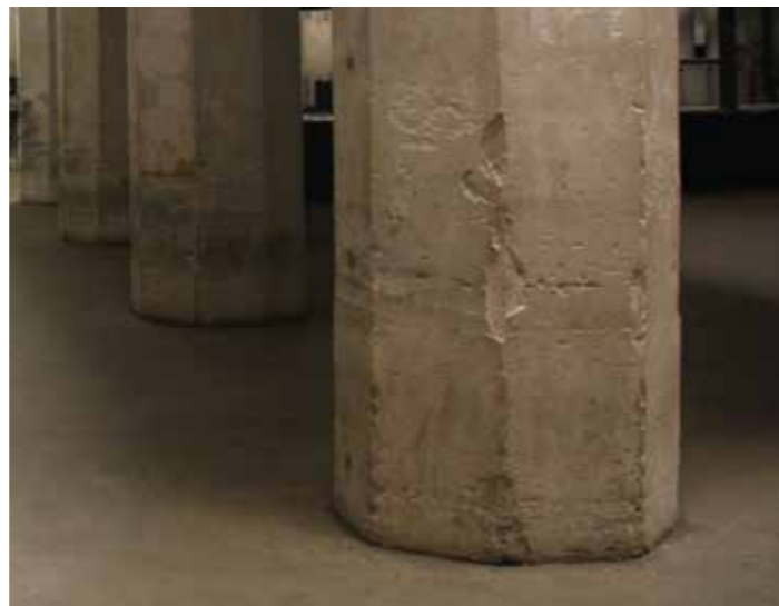
Lower parts of concrete columns and surrounding walls still carrying traces of the machines movement
