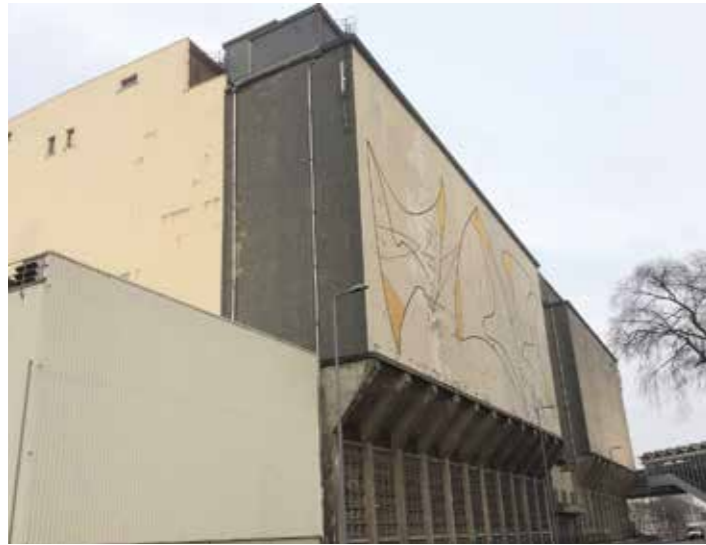
Exterior - west façade
