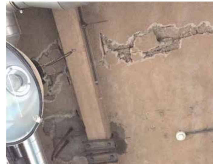
Interior - ground floor ceiling
