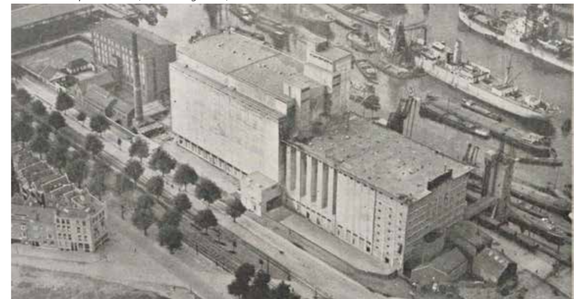
south facades phase 1 & 2 (1931 de Ingenieur)
