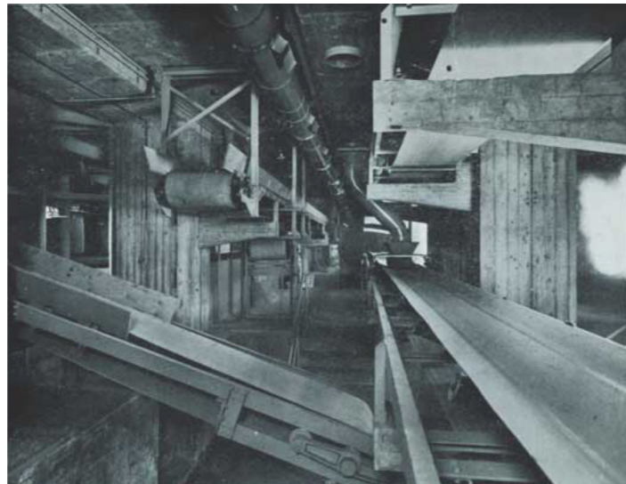
conveyor belts in the basement, Transformers report, p.27
