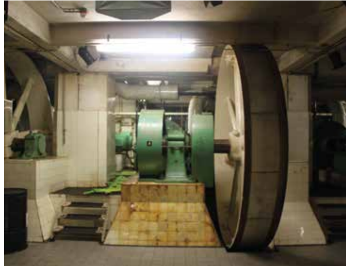
Electro-motors with flywheels which power the pneumatic pumps they were cooled by cooling pumps which used water of the Maashaven. These motors really give meaning to the basement as to what it function was.
