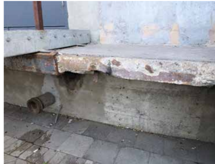
Exterior - north façade
