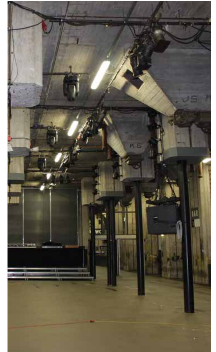
construction work finished phase 2
