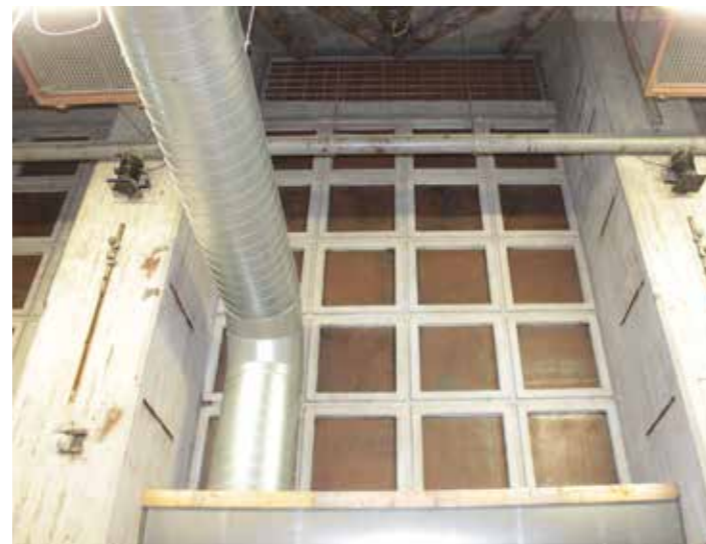
Current - interior The plofroosters are closed off with metal plates on the inside.
