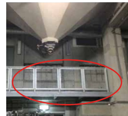
Current - interior Original windowframes remain visible in front of / on the surface of new concrete filling.
