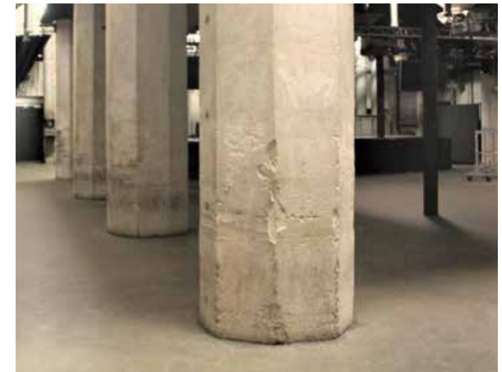
Interior - ground floor column
