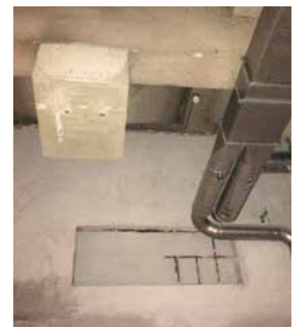
Current - interior Original windowframes remain visible in front of / on the surface of new concrete filling.
