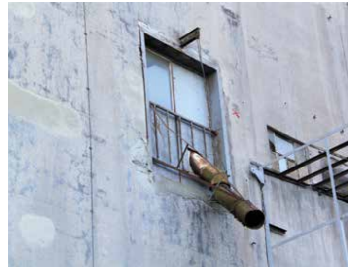
Exterior - north façade
