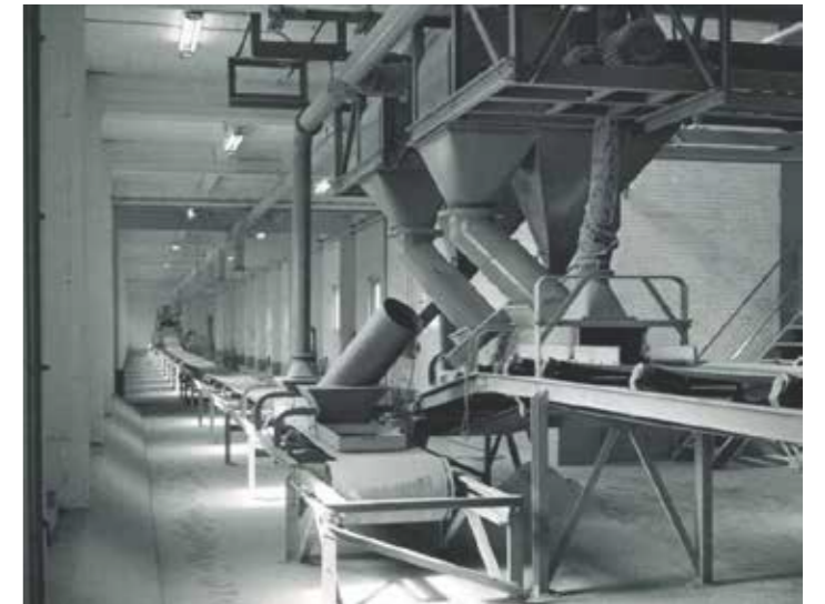
conveyor belts in the basement, Transformers report, p.72
