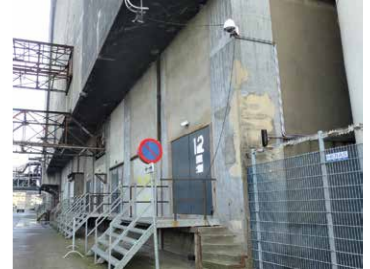
Exterior - north façade
