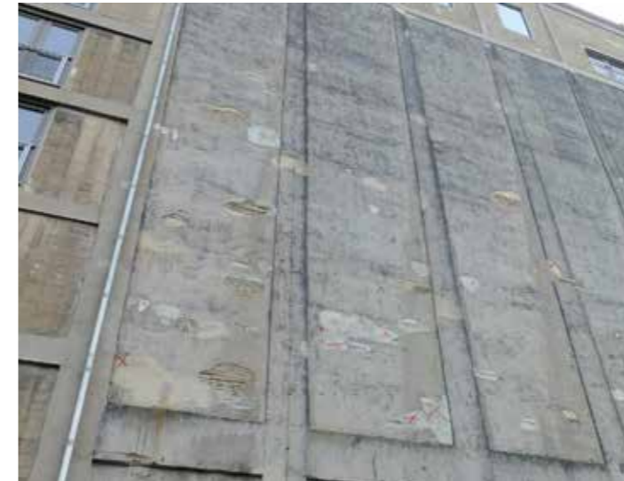
Exterior - north façade
