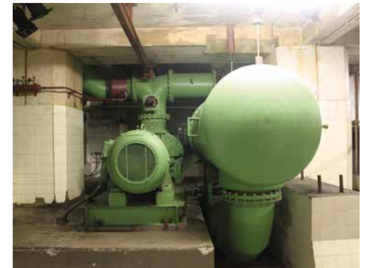
Pneumatic pumps which create a vaccum (suction) which make it possible for the elevators and cranes outside to suck 400 tons of grain out of the boats per hour and transport them indoor. the machines were made by SIEMENS
