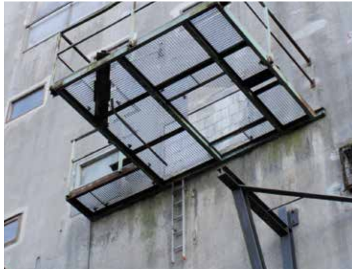
Exterior - north façade
