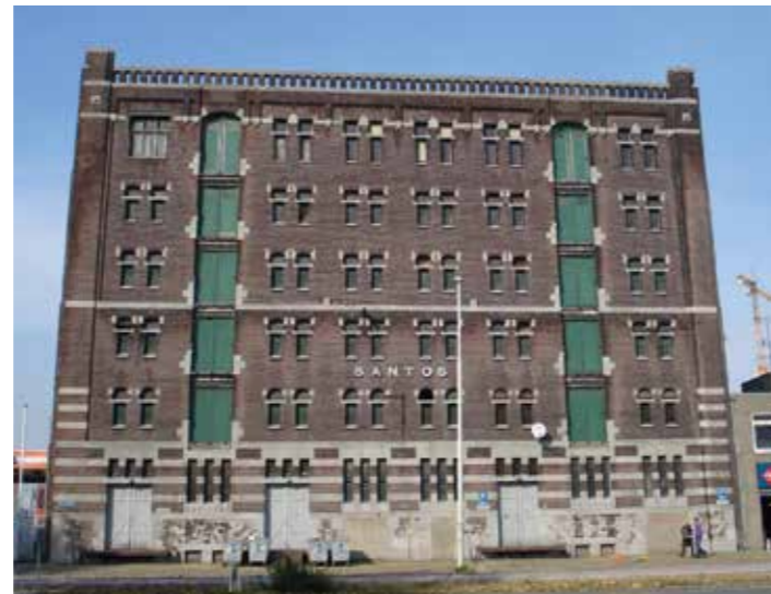
Santos warehouse. Design by Stok for Blauwhoedenevem. Built in 1903. source: http://rijksmonumenten.nl/monument/513940/pakhuis-santos/rotterdam/
