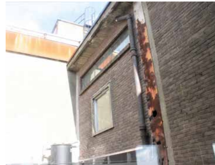
Exterior - west façade
