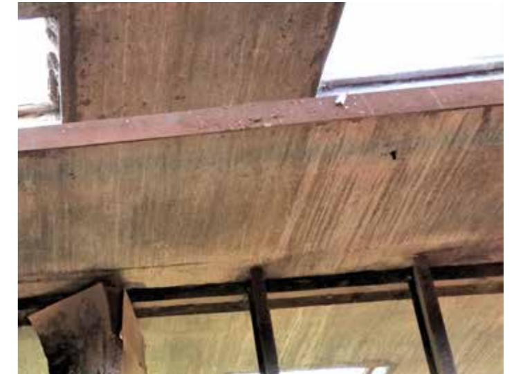
Interior - north façade, tower, 7th floor
