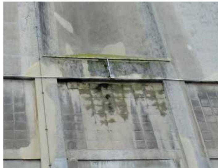
Exterior - north façade
