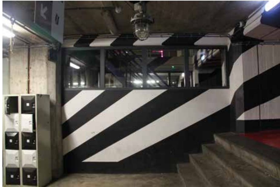
New paint stripes throughout the basement of the second phase/ Brinkman to make a contrast between the existing rough surfaces of the bare concrete and the newly painted surfaces which highlights the texture differences.
