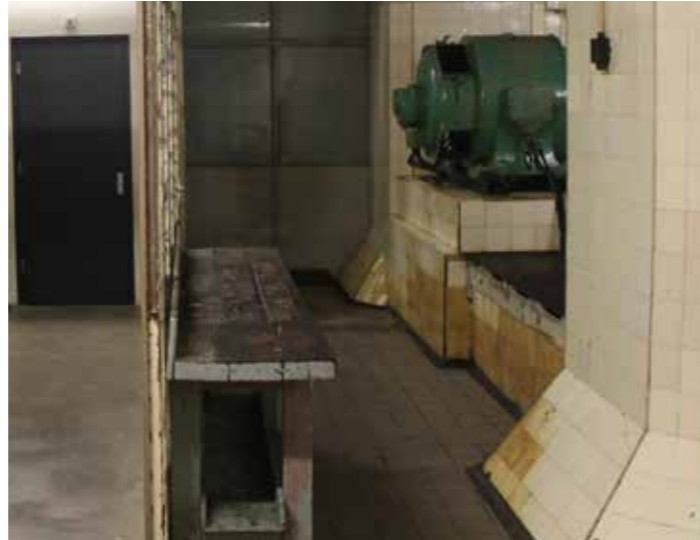
Objects adjacent to the former conveyor belts still present in the basement
