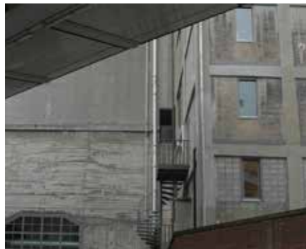
Drainage system in the 1st phase is rationally positioned at the edges of the roof and extended to the corners of the building, as well as the sides of the silos
