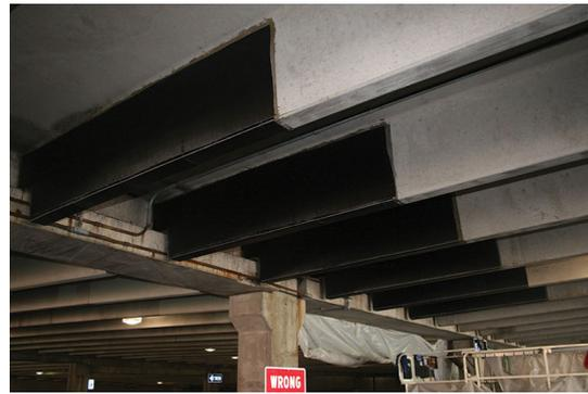
(b) U-shaped FRP laminate applied on concrete beam [4]
