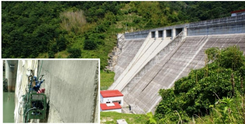
**Figure 2.9:** Dam in Japan strengthened using SHCC [36]
