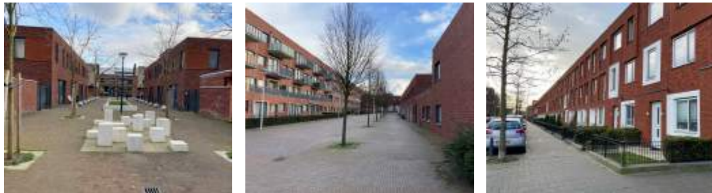
Figure 16. The newly constructed private houses, built in 2000, locates in the middle of Morgenstond, near Leyweg shopping center.
